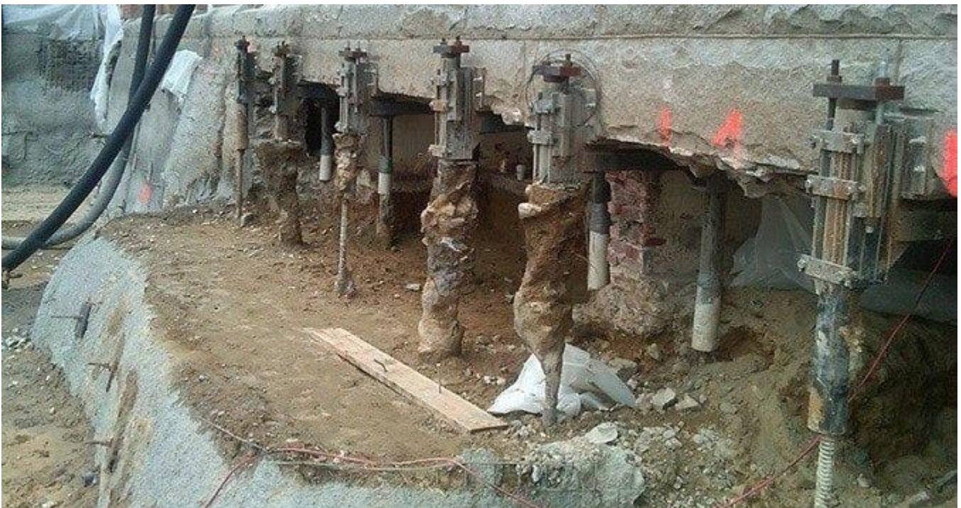
Fig.1: Underpinning Method; Image Courtesy: Moretrench -Hayward Baker Company
