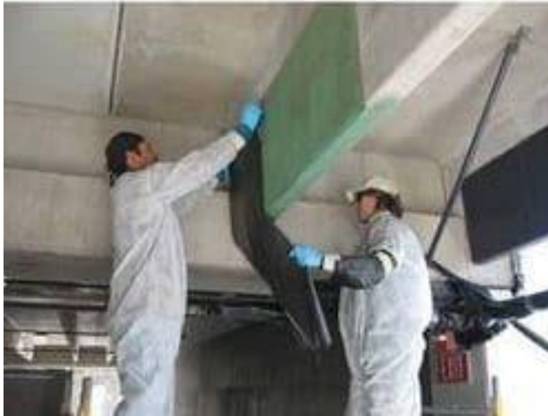
Fig. 3: Retrofitting with FRP Composite
