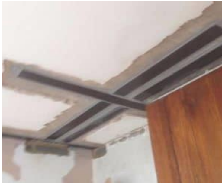
Fig. 5: Plate Bonding
