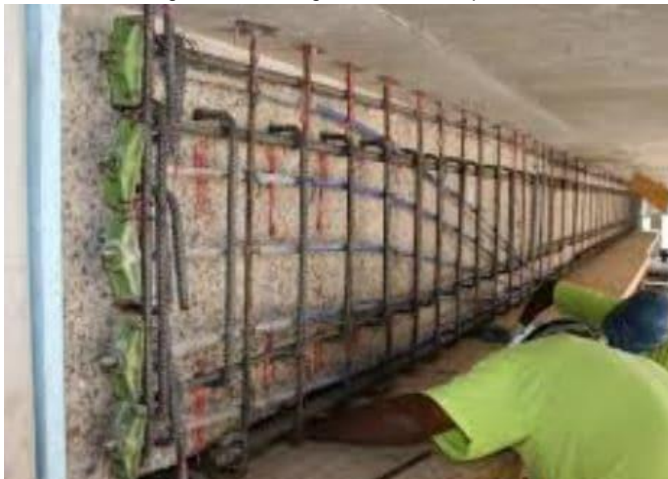
Fig. 4: Section Enlargement
