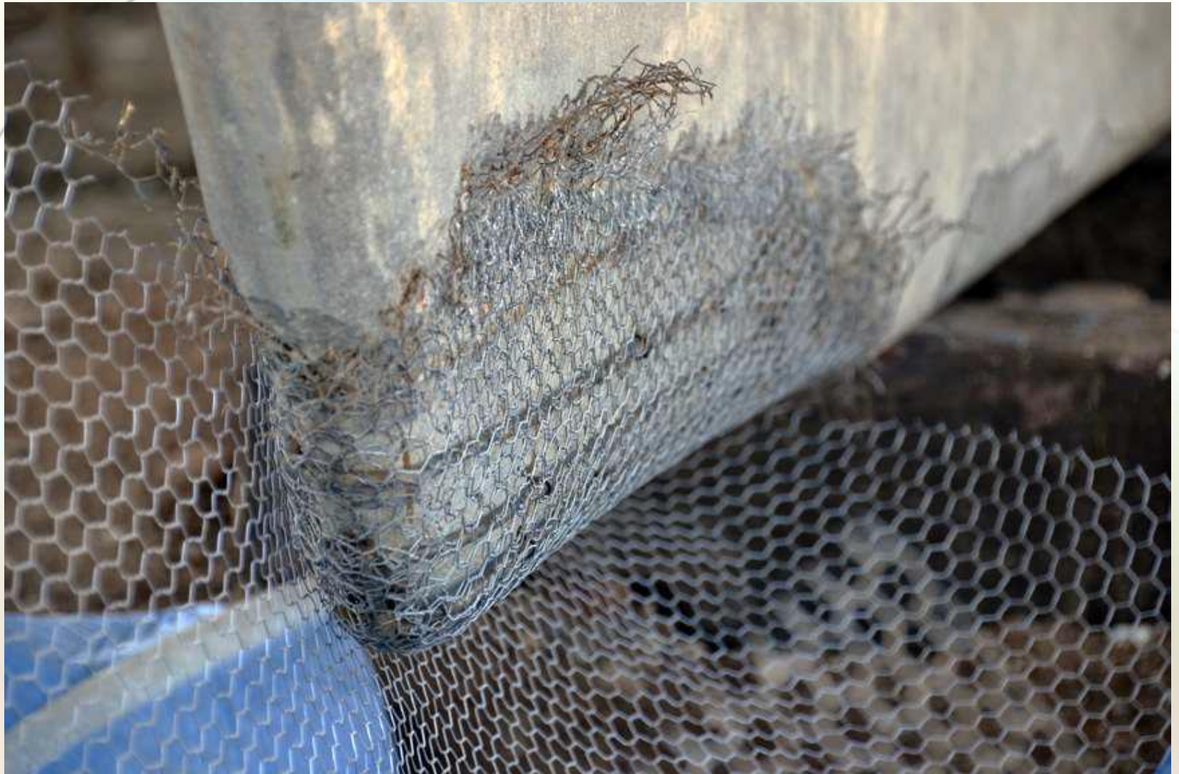
TYPICAL CROSS SECTION OF FERROCEMENT
